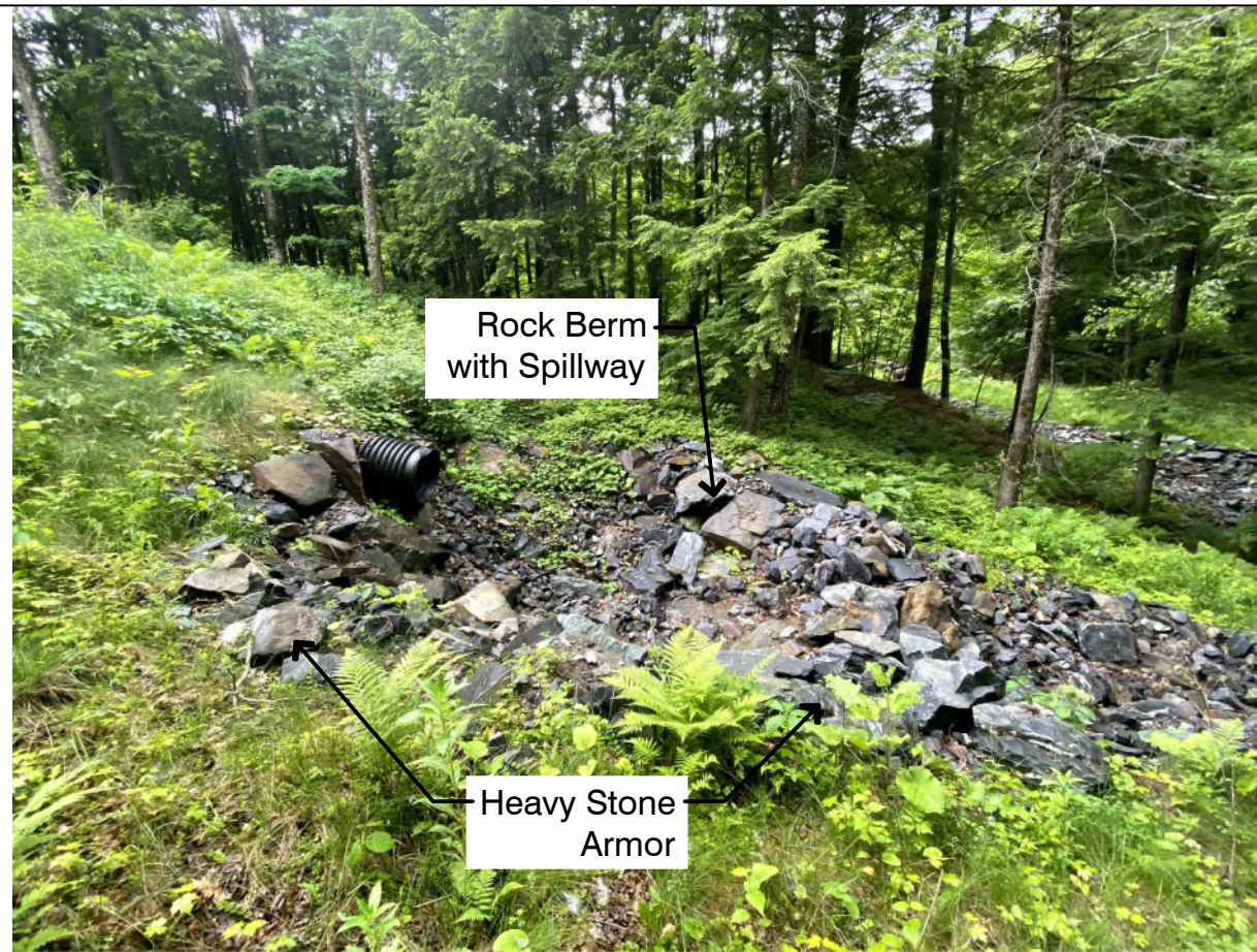
Photo 2. Example of Stone Splash Bowl Outlet Protection
